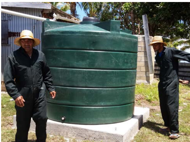
Water tank is installed as near as possible to the house and the water tap facing the main door for easy access.
