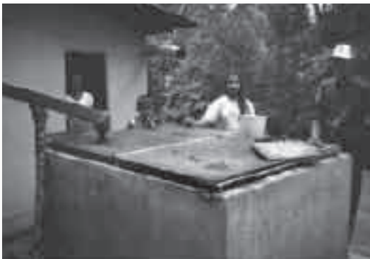
A concrete storage
