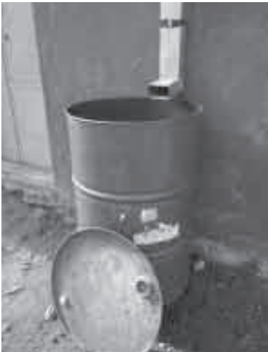
Rainwater collection in a barrel.
