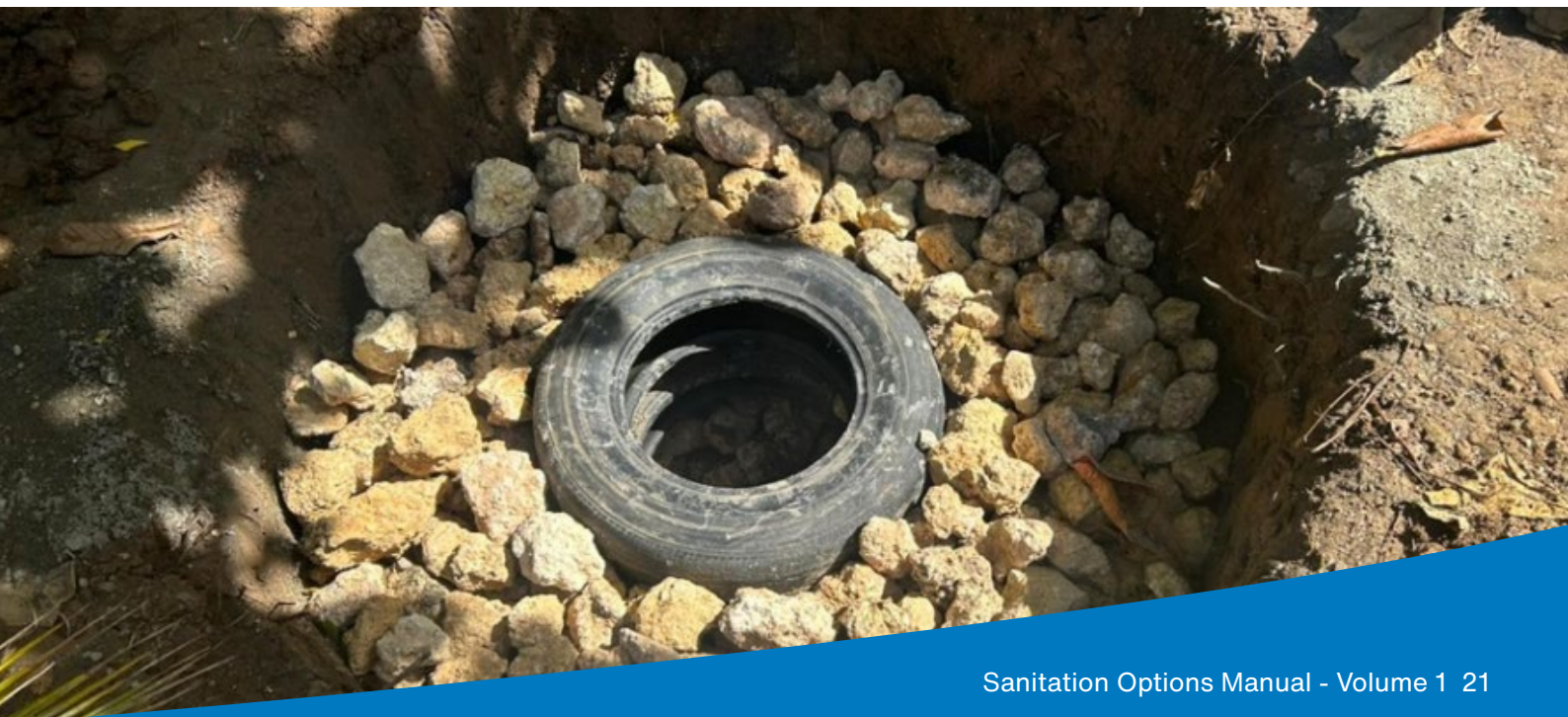
Figure 5. Typical Cesspit arrangements – 'direct' and 'offset'
